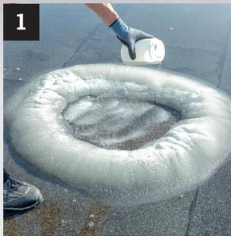
Sprinkle the granulate directly into the standing water around the work area. A gel forms. A solid dam, which reliably keeps back the water is formed within only 3–5 minutes. If necessary, sprinkle more granulate in the work area.
